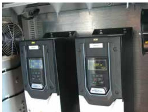
Flygt SmartRun intelligent pump controllers reduce system clogging with automatic sump cleaning and pipe flushing functions.
