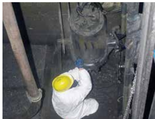
The traditional system required intervention up to three times every week.
