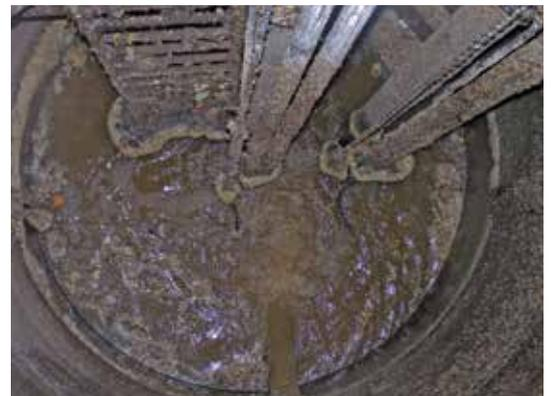
As well as a heavy flow of wastewater, the station also takes in storm water, often including large quantities of solids, which led to frequent clogging issues.
