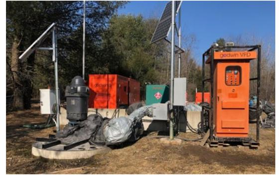
The powerful hydraulic design of the Goulds Water Technology vertical turbine pump provides the lift and flow-rate needed to achieve this site's maximum withdrawal rate.
