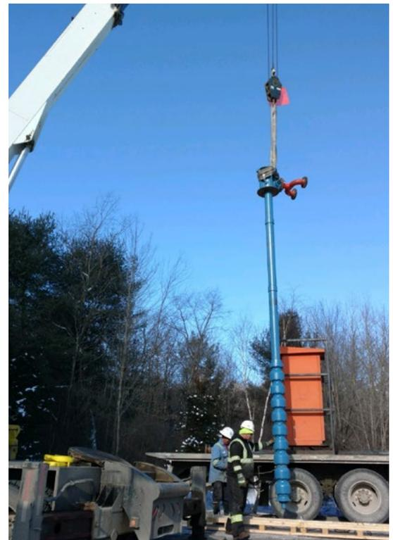
Xylem's field team installed high-lift Goulds Water Technology vertical in-line turbine pump down into the well shaft with a connected Godwin variable frequency drive and MJK flowmeters provided greater visibility.
