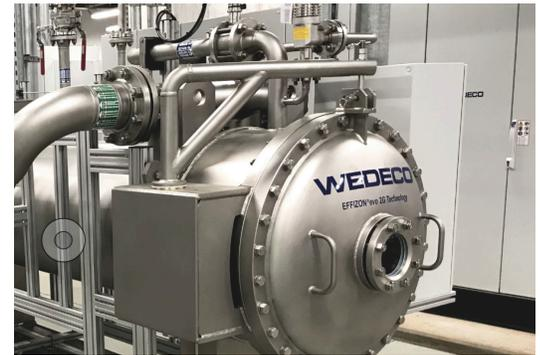
The Xylem-designed AOP system consists of two Wedeco PDOevo 900 ozone AOP systems, each producing 1,000 pounds of ozone per day.
