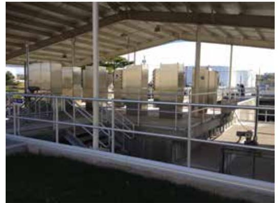
Stainless steel air conditioned ballast cabinets supply the power to the UV lamps
