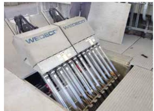
Inclined orientation and high power Ecoray lamps make for a small footprint, reducing construction costs
