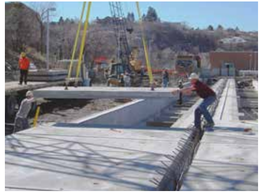
Construction of the ozone contact chambers
