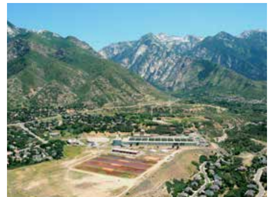
Aerial view of the Little Cottonwood Water Treatment Plant
