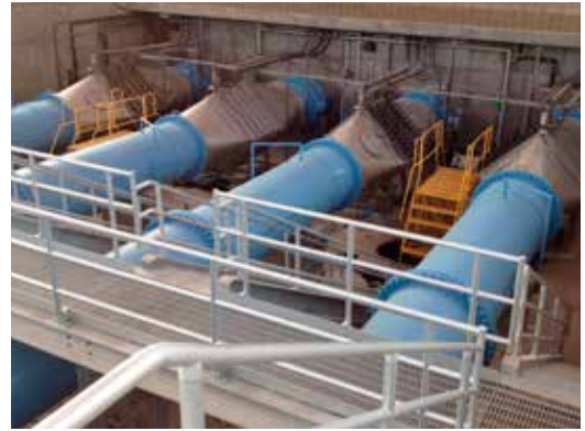
Four Wedeco K143 Series UV reactors shown in parallel
