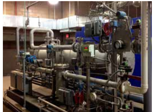
Wedeco PDO evo 7000 skid mounted ozone generator
