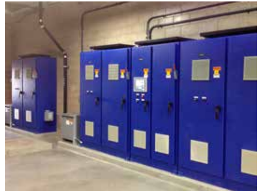
K143 Series UV power supply remote enclosures
