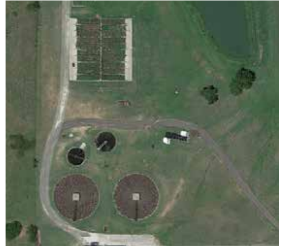
Perry WWTP view before dewatering project.
