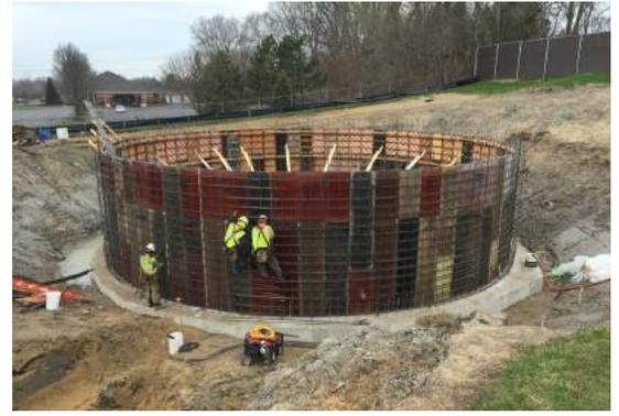
Crews install rebar on a tank during the expansion of the Zeeland Clean Water Plant.
