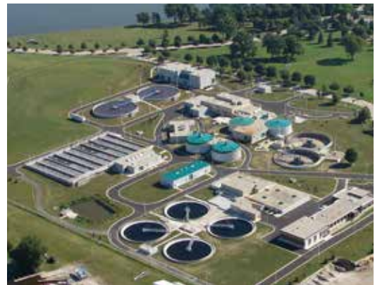
Renovations allowed the Fond du Lac WWTP to double hydraulic capacity.
