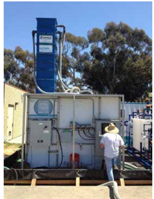
Xylem’s Leopold Oxelia ozone-enhanced biofiltration System
