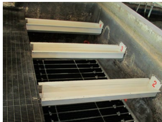
New Type S ® Underdrain with I.M.S. ® 200 media retainer.
