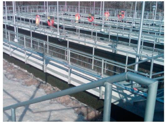
These seven deep bed filters are 89' long x 13' wide and provide Enhanced Nutrient Removal. Effluent nitrate is <0.5 mg/L and effluent phosphorus is <0.2 mg/L.
