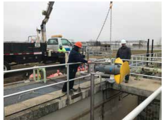
Installing the 4320 mixer
