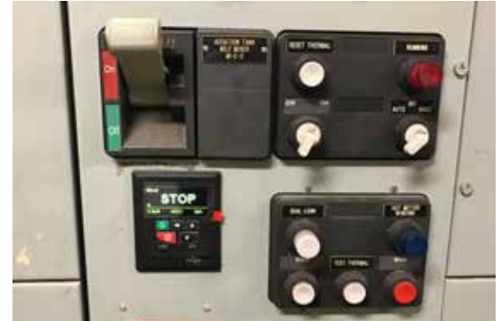
Mixer control fits easily onto existing panels - showing “STOP” during installation
