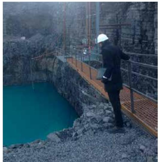
The Flygt 4680 submersible mixer displaced warmer water from the bottom of the quarry to the surface, preventing ice formation.
