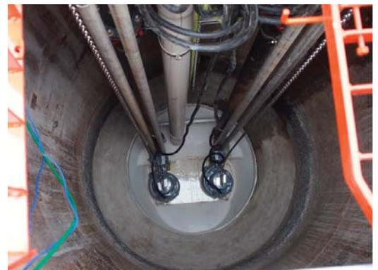
The wet well with two Flygt submersible pumps and TOP 150 insert
