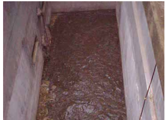
A view of the FOG layer being re-incorporated into the influent after the Flygt mixers were started.
