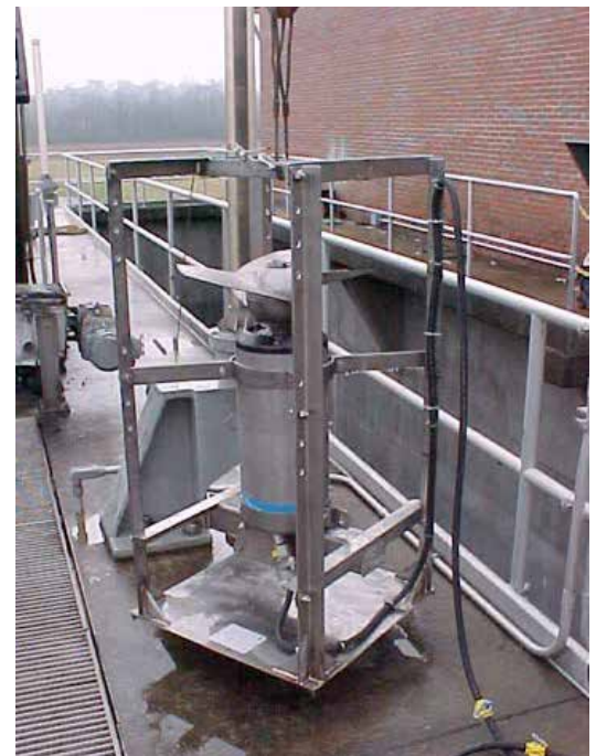
One of the two Flygt SR4660 mixers waiting for installation.
