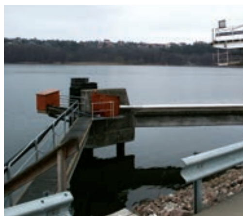
Connection points located alongside the quays enable the ferries wastewater to be transported to nearby Flygt pump station.
