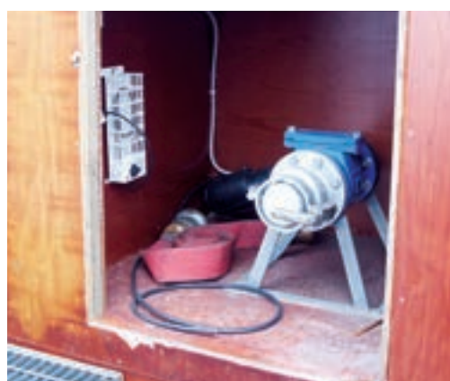
Connection points located alongside the quays enable the ferries wastewater to be transported to nearby Flygt pump station.
