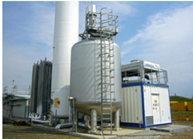
The ozone plant consists basically of the components ozone production, LOX storage tank, ozone dissolution in wastewater, ozone reaction and degassing tank, air cooled chiller unit and residual ozone destruction.
