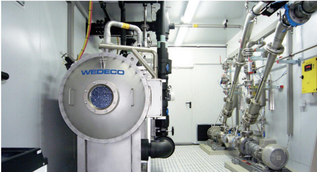
The WEDECO PDO 2500 Ozone Generator (left) and the pump-injection-system are housed in an insulated container, perfectly fitted for the installation of a large scale ozone system. This completely preassembled system reduces onsite installation effort and makes concrete housing redundant.
