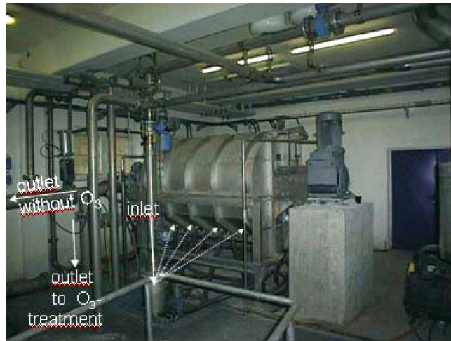
Pressure disk filter
