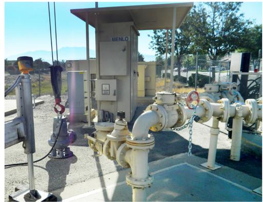
The Flygt 3102 electric submersible pump about to be lifted into position in the wet well.
