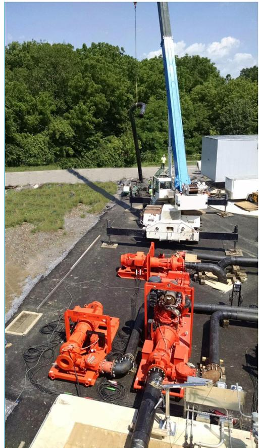
The Godwin HL250 pumps and piping were moved into place by crane.
