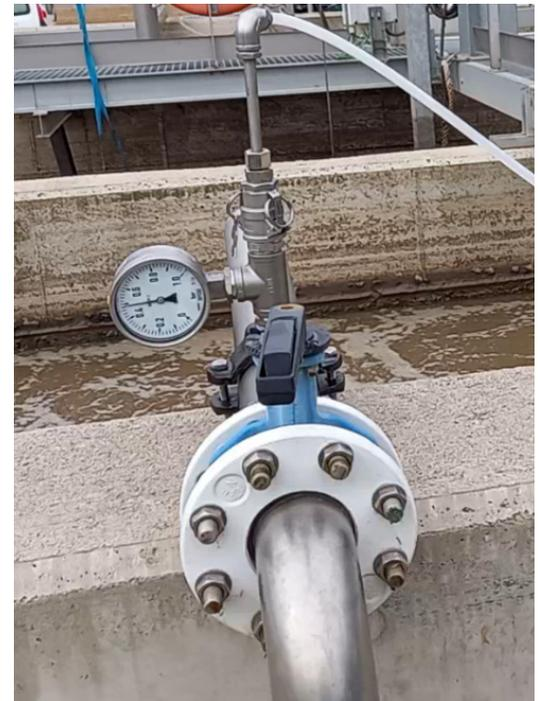
The accessories of the cleaning kit were mounted on the pipe collar. A pressure gauge was also installed to monitor the cleaning progress.
