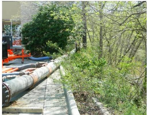
The discharge pipe was designed to flow behind a local business, so we avoided shutting down their only access to their service bays. The pipe was held in place on the steep bank with slings and binders. Trees helped support the weight of the pipe to prevent it sliding toward the creek.
