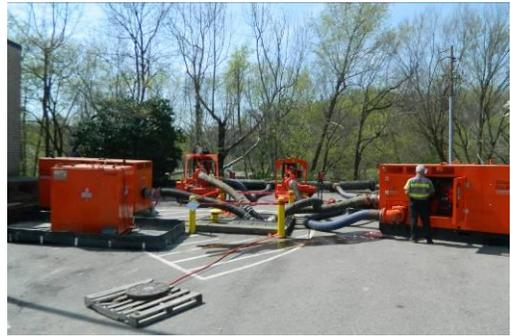
Pumps were placed around an existing siphon box, which was used as a suction point.
