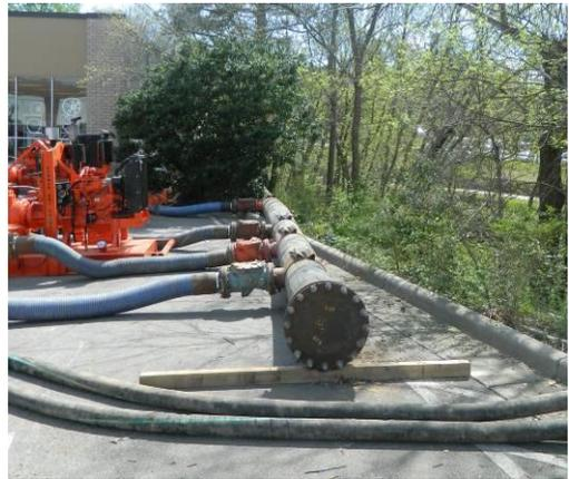
To save time, four saddles were mounted to the discharge line for ease of installation and to minimize setup time.
