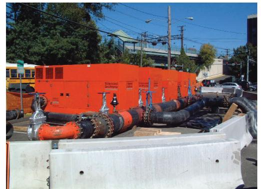
Twenty Godwin pumps were on site for the duration of the project. Because of the size and quantity of pumps required, the town opted to rent the equipment to save transportation, storage and maintenance costs.
