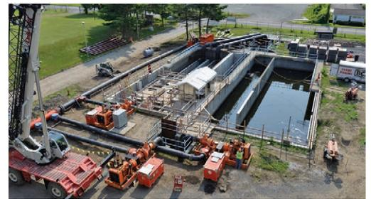
The temporary bypass system allowed Albany County and BCI Construction to reduce the footprint of its wastewater treatment plant upgrades.
