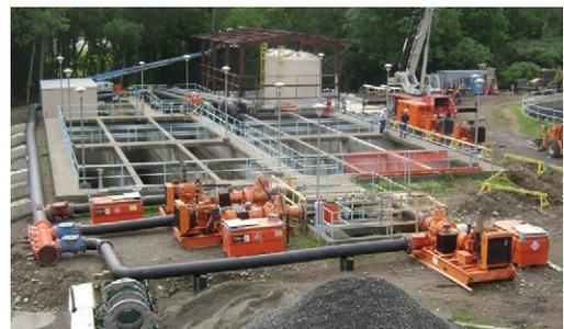
The Albany plants were outfitted with three CD400M 16-in. Dri-Prime Pumps each. Godwin Heida 750AX Axial Flow Dewatering Pumps were also added; all equipment was rented by the county for the project.
