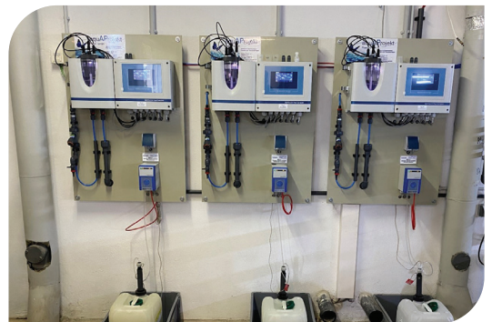
Three analyzers & controllers DEPOLOX Pool Compact
