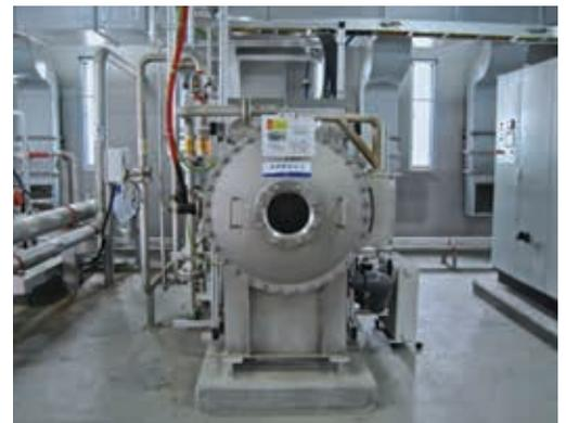
Three WEDECO PDO 1000 ozonators are producing up to 51 kg of ozone per hour from liquid oxygen.
