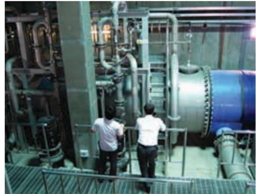
Two ozone injection lines with a flow rate of 17,000 m<sup>3</sup>/h each.
