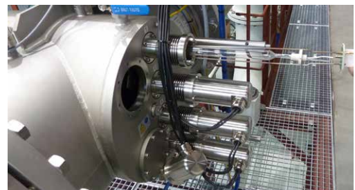
UV lamps and sensors are accessible from one side and can be replaced quickly and easily without having to empty the reactor.
