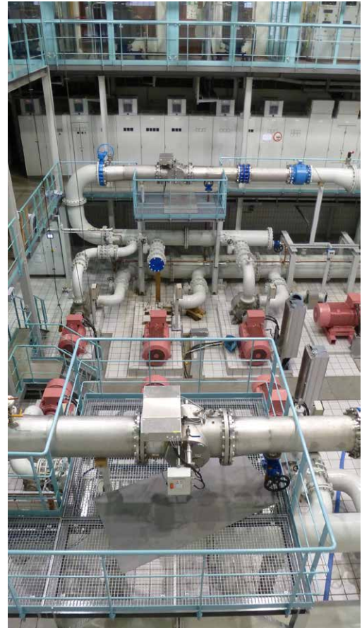
UV reactors were retrofitted and installed above the mains pipe.
