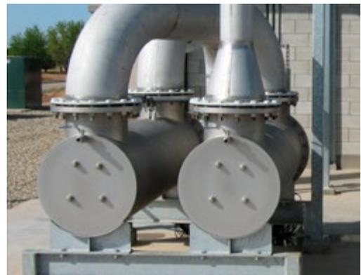
One of four trains (three duty and one standby) in the system. Each train is designed to disinfect one to two million gallons (< 7,570 m<sup>3</sup>) of water per day to the stringent California Title-22 water reuse standard.
