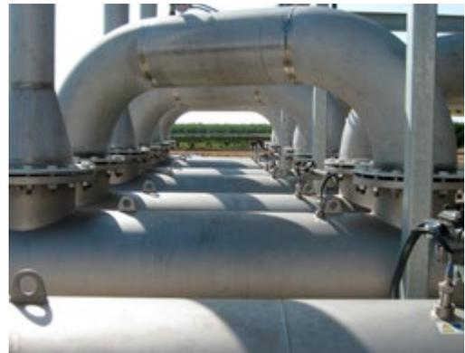
Each reactor is equipped with an internationally recognized ÖNORM compliant UV sensor which allows for active monitoring of UV performance. The sensors enable the automatic control mode to adjust UV lamp output to the actual level needed to meet the required 80 mJ/cm<sup>2</sup> NWRI dose using minimum energy.
