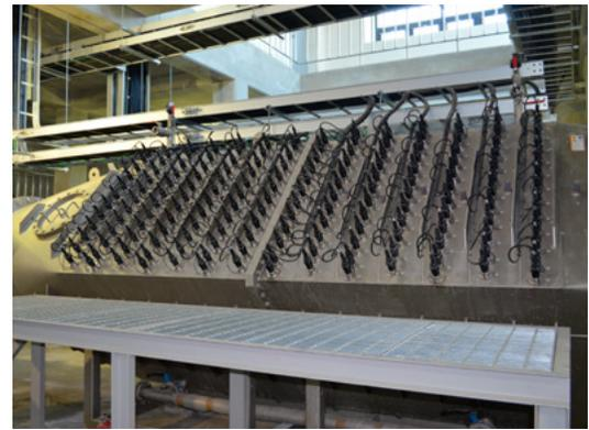
The Wedeco MiPRO photo K-Reactor has a staggered lamp arrangement for highest flexibility and dose distribution.
