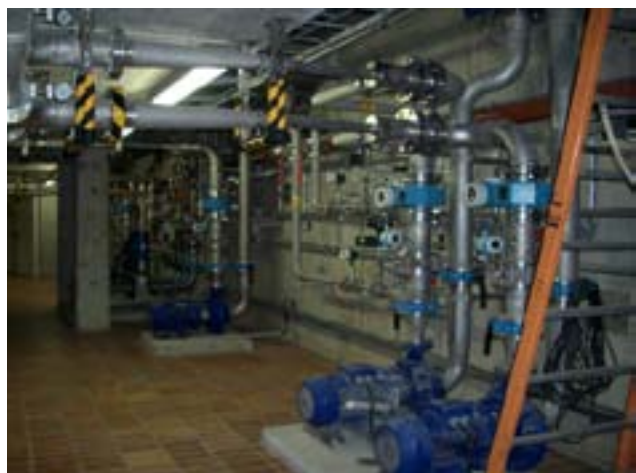
Ozone injection system during installation
