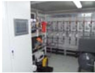
Containerized WEDECO SMO/SMA Ozone generator with gas distribution.
