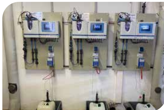
Three analyzers & controllers DEPOLOX Pool Compact
