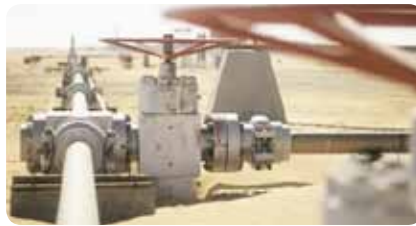
Industrial use , such as cooling water and process water in the petrochemicals, pulp and paper, steel and textile industries.
