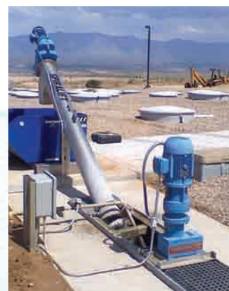
The SPIRALIFT SL with grinder is installed at the newly designed wastewater facility in Arizona.
