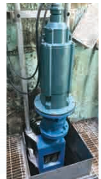
This grinder is utilizing a submersible (IP68) motor.
