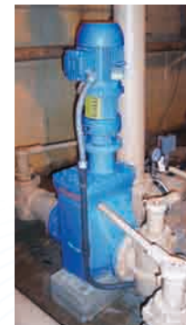
A TASKMASTER inline grinder with flange housing.
