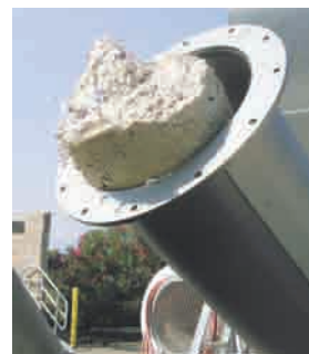
The discharged solids are cleaned and compacted.
