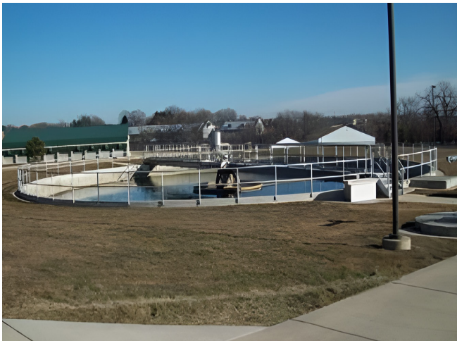
Fig. 7, A photo of Watertown WWTP
