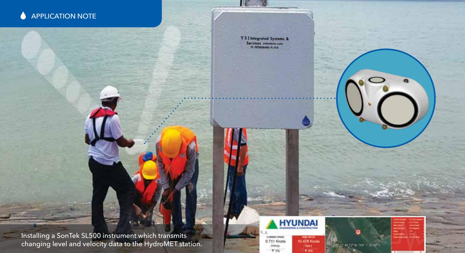
Installing a SonTek SL500 instrument which transmits changing level and velocity data to the HydroMET station.
