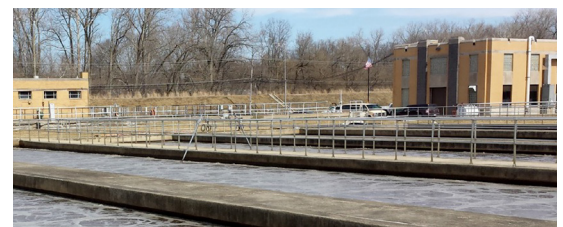
Muncie, Indiana, Water Pollution Control Facility
