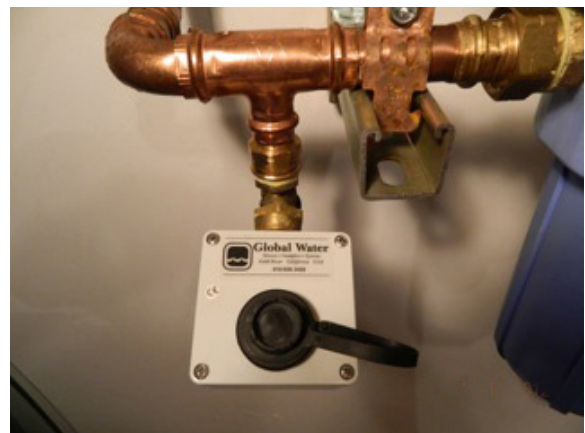
The PL200-G Pressure Logger's garden hose connection and compact, water-resistant enclosure makes it easy to use and mount anywhere.
