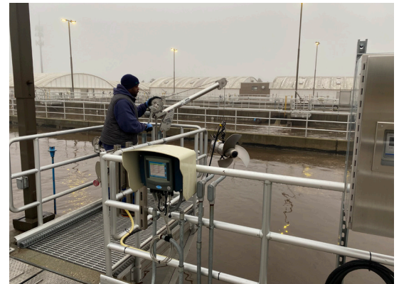
A facility operator pulls a Flygt 4220 adaptive mixer for inspection.
