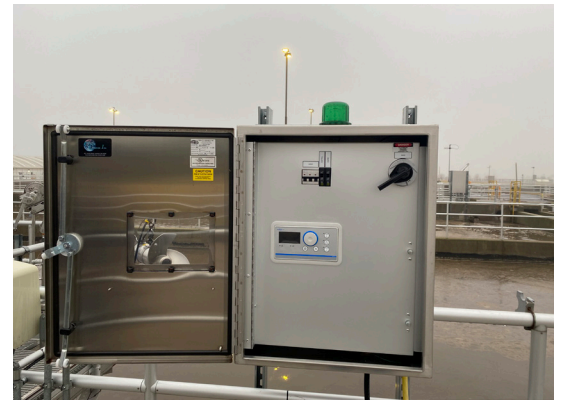
Integrated advanced controls allow the adjustment of thrust and energy consumption to adapt to process changes as well as providing continuous communication with the operator.
