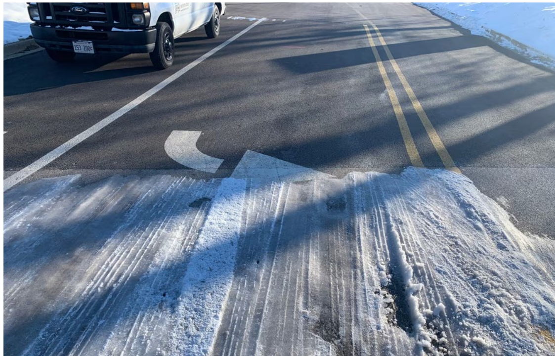
WarmlyYours installed two heated driveways for a temple in Chicago, ensuring that their community could come to worship without fear of icy roads. IMAGE COURTESY OF WARMLYYOURS
