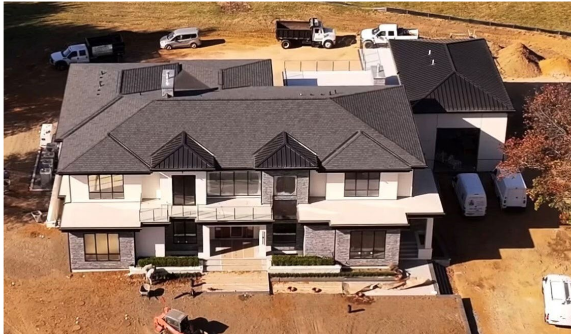
NextGen was involved with a 15,000 sq. ft. custom home that featured a comprehensive radiant system. PHOTO COURTESY OF NEXTGEN PLUMBING, HEATING & COOLING
