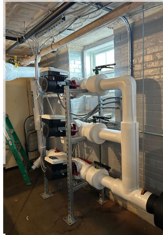
Xylem's hydrovar® X-enabled smart pumps were selected for their compact design, intuitive programming and ease of serviceability.
