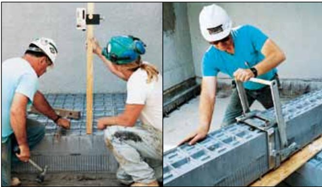
Installation is easier with Type S Technology Underdrain because blocks can be set to level  $\pm 1/4$  inch (left). Assembly of laterals is easier because the blocks simply snap together to form leak-resistant, distribution efficient laterals (right).
