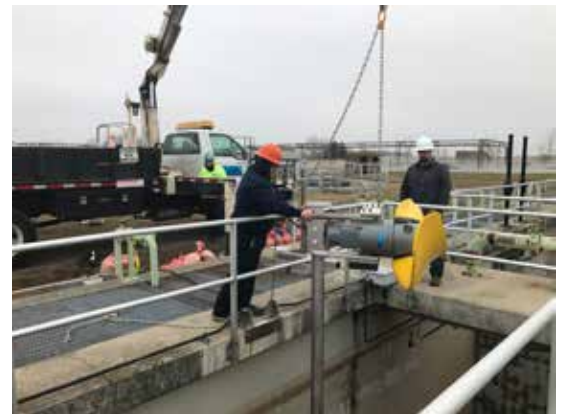
Installing the 4320 mixer
