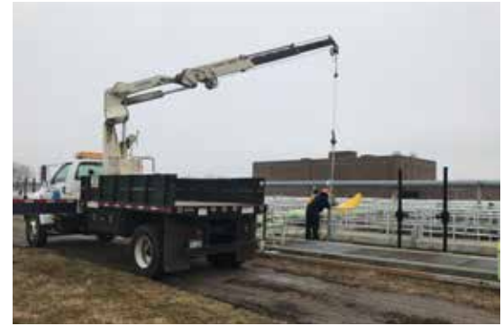
Submersible mixer drops in easily from truck to tank
