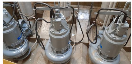
Buckeye Pumps equipped the pump station with three Flygt NP3531 20” units, each with 130 HP closed-loop cooled motors.
