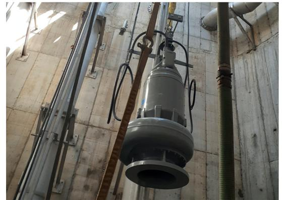
The Flygt deep lift mechanism helps simplify installation and maintenance when needed, eliminating the need for personnel to enter the wet well.
